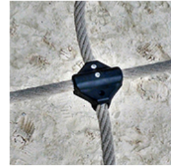
Poly Fix With Missing Screw
