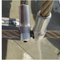
Ferrule T With Loose Screw
